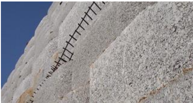
Retaining wall built for an attenuation pond.
