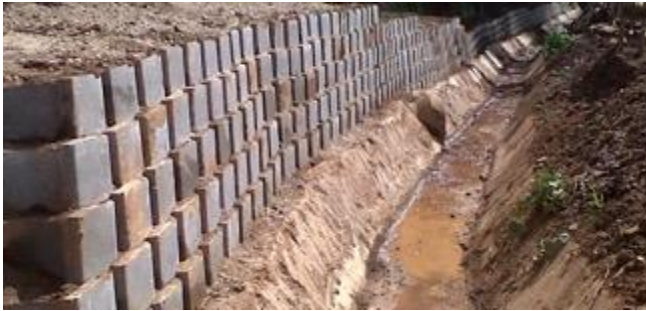
Retaining Wall built next to the water channel.
