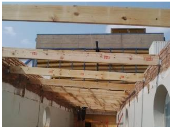
Installation of roof beams.
